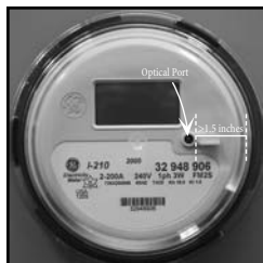
Electronic Meter Measure the distance between the FRONT optical port and the outer rim of the dome. It should be NO LESS THAN 1.5 inches (37 mm). Use Quick Install Guide or see section 5.3
